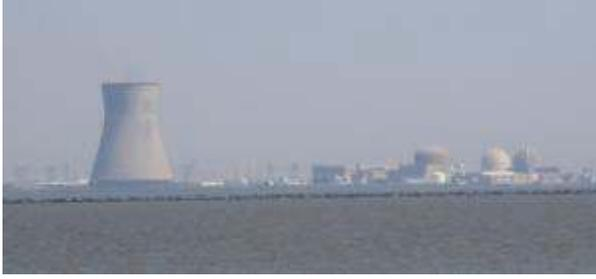
Under NRC guidelines, Salem and Hope Creek had to shut down if there were sustained winds of 74 miles per hour or the river reached 99 feet in depth. The plants' "design basis" states the sea wall would repel water up to 120 feet, a level only anticipated with a Category 4 hurricane.
